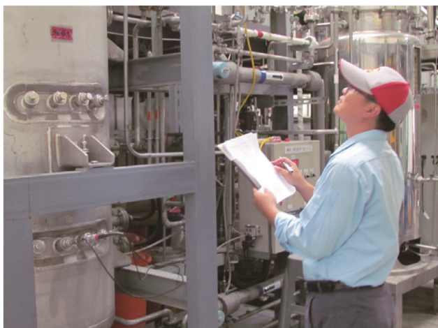
R&D Team Members Regularly Check The Fermentation Tank.
